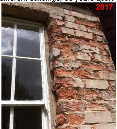
Impermeable coatings result in trapped moisture and building decay
